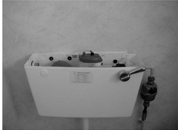
**Figure 5 Fitted Ecoflush**
