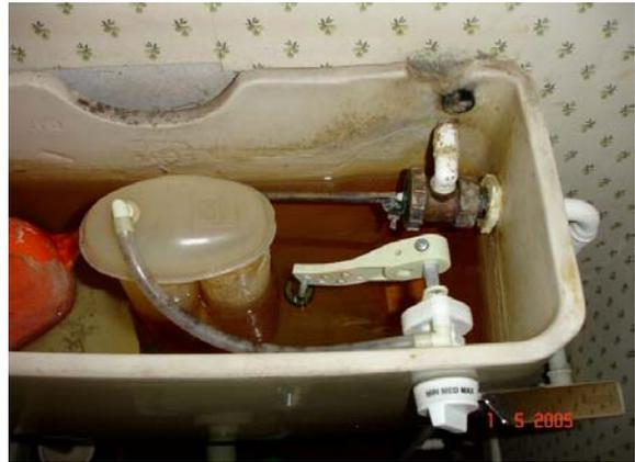
**Figure 7 Fitted Variflush A**
